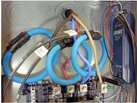
PowerScout 3+ w/RoCoil CTs attached to load
