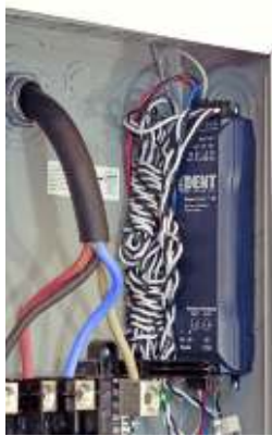
PowerScout 3 mounted within electrical panel
