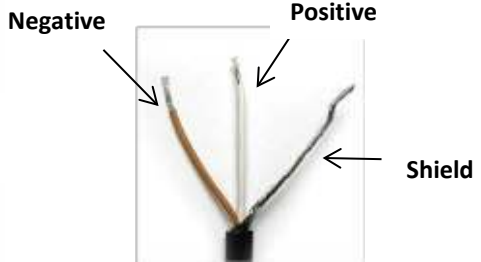
Shield Wires from DENT RoCoil CTs connected to ELITEpro SP
