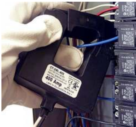
Photo 2: Install CT Around Conductor.
