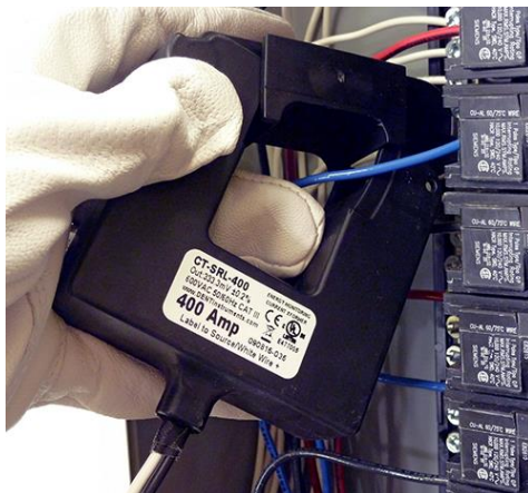
Photo 2: Install CT Around Conductor.
