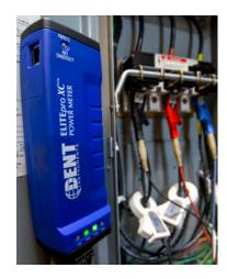
**Above:** An ELITEpro XC meter installed at the job site by Roger's Machinery to capture the energy consumption of a compressor system.
