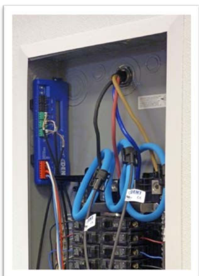
PowerScout 3037 w/RõCoil CTs attached to load
