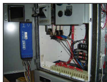
Figure 3: In addition to being rugged and reliable for use by non-expert operators, the ELITEpro SP instruments are compact enough to fit inside most electrical panels.
